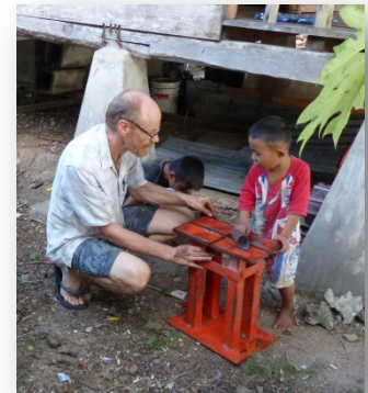
Some eager helpers cleaning up the concrete block moulds
