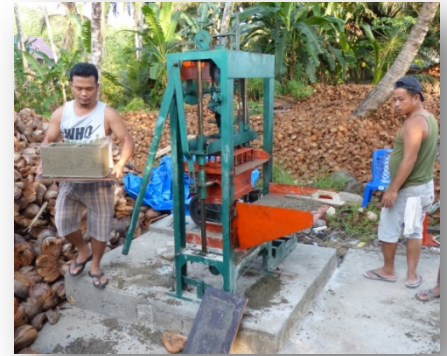
Matt making a concrete block with the new block machine
